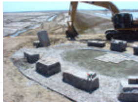
Memorial under construction by MES Poplar Island crew
