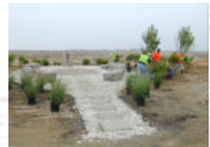
Memorial grounds under construction by MES Poplar Island crew
